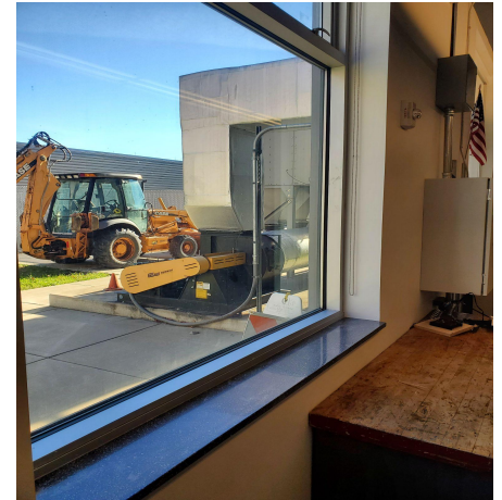
Central to dust collector and outside wall for venting of machines.
